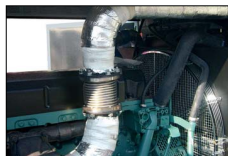
Compensatore gas di scarico Exhaust gas compensator Compensateur d'échappement Junta flexible para escape
